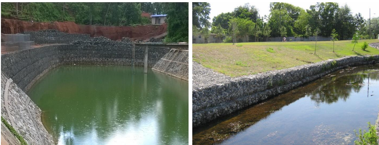
Fig. 125 Gabions for Ponds Protection
