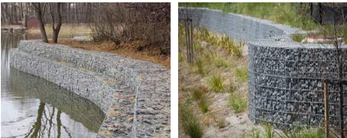
Fig. 124 Gabions for Drains and Rivers Protection
