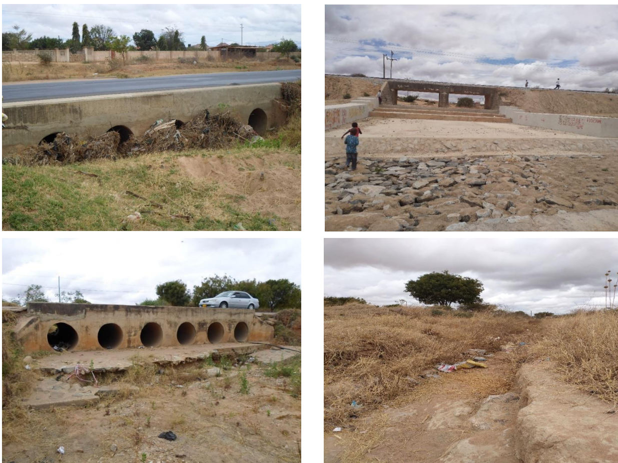
Fig. 20 Kisasa Storm Water Drain
