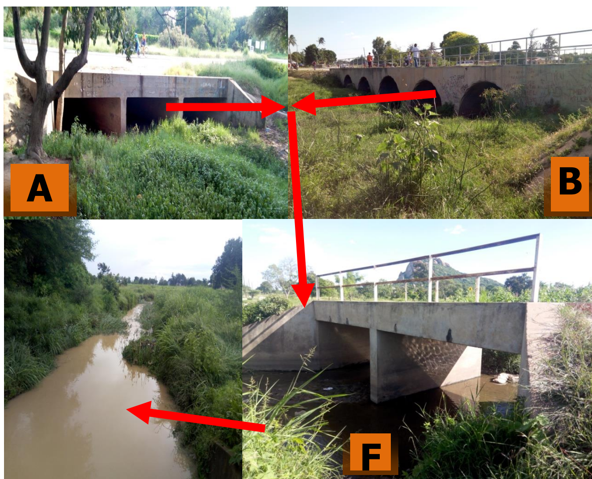
Fig. 34 Culverts A from Area D, B from Kikuyu and F in Mlimwa C
