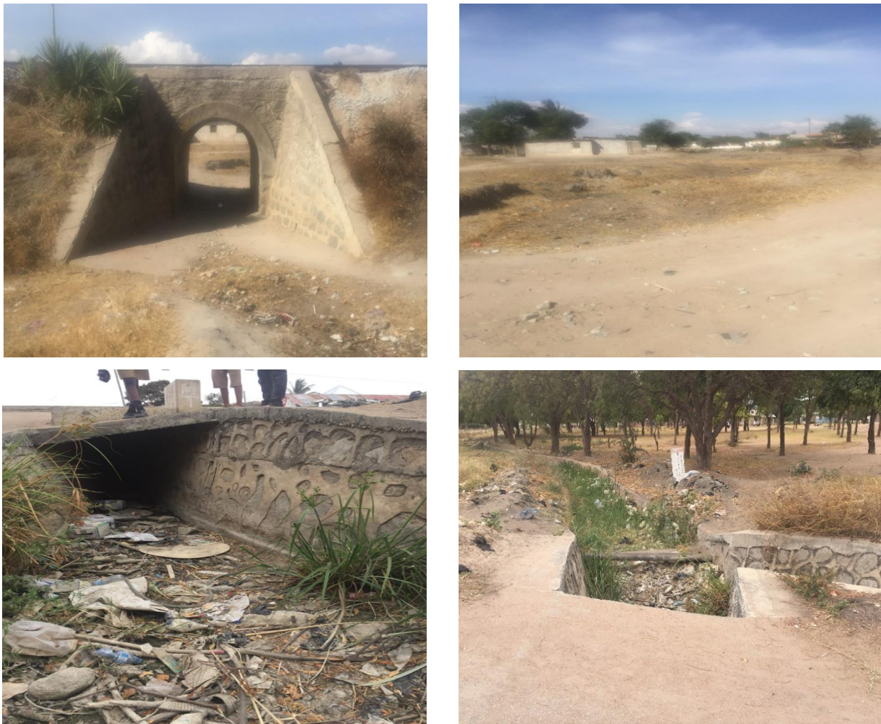
Fig. 15 Kizota Storm Water Drain
