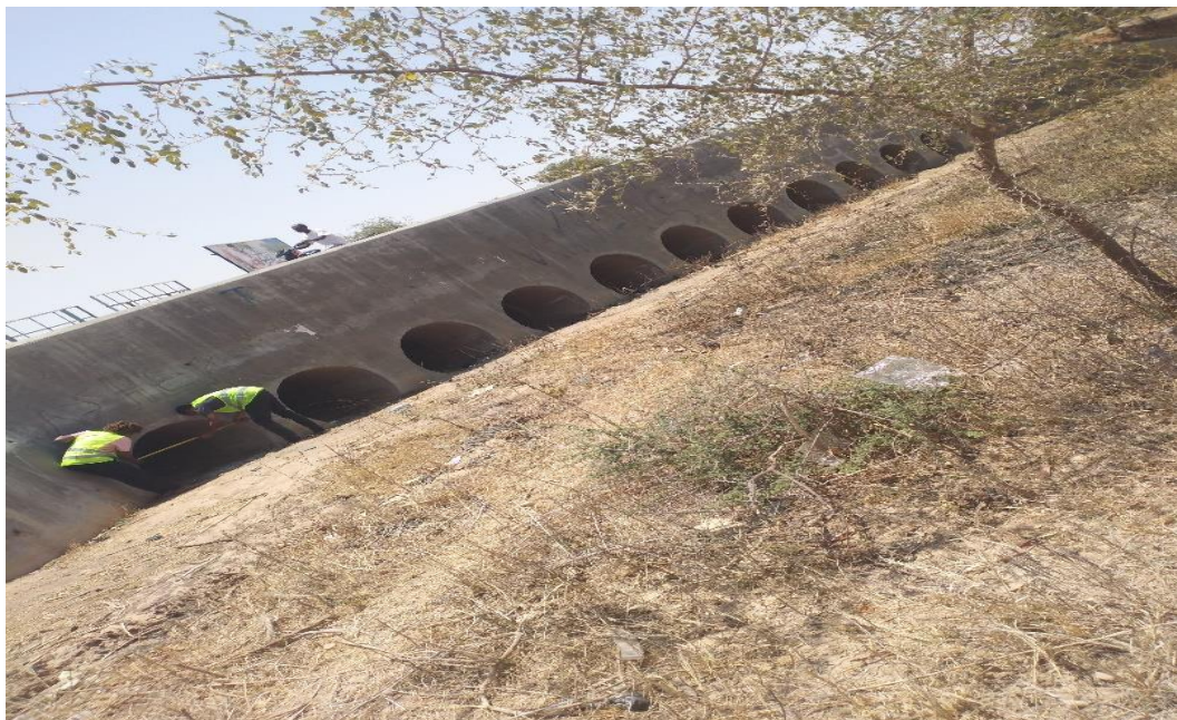
Fig. 25 Mkalama-Tambukareli Storm Water Drain
