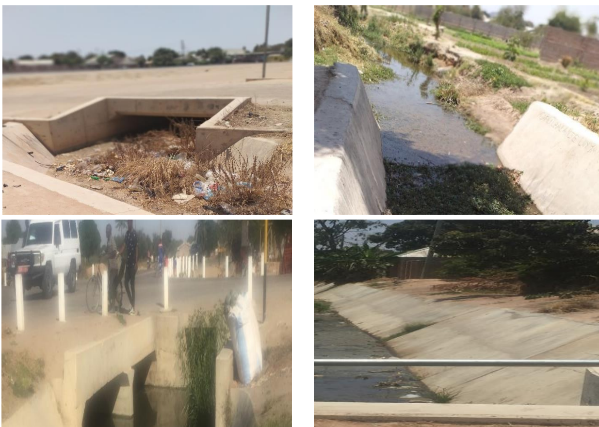
Fig. 16 Nkuhungu Storm Water Drain
