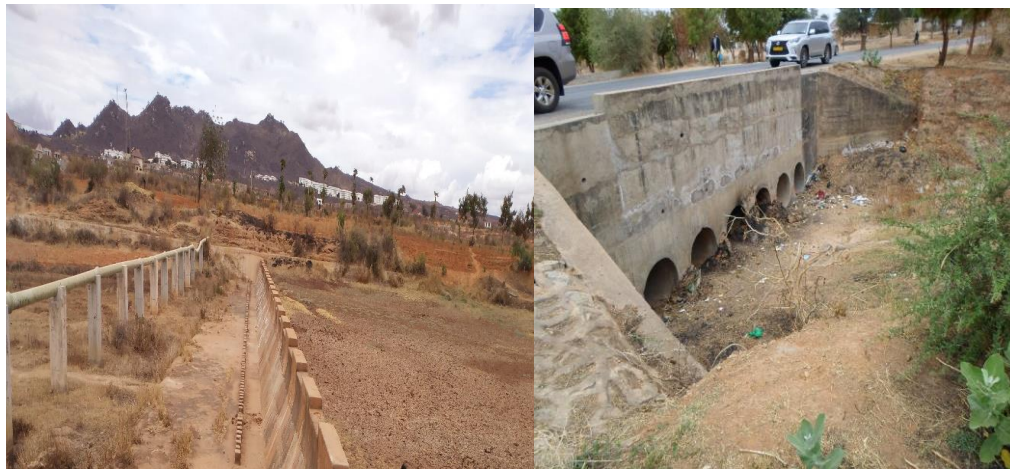
Fig. 24 Mkalama Storm Water Drain
