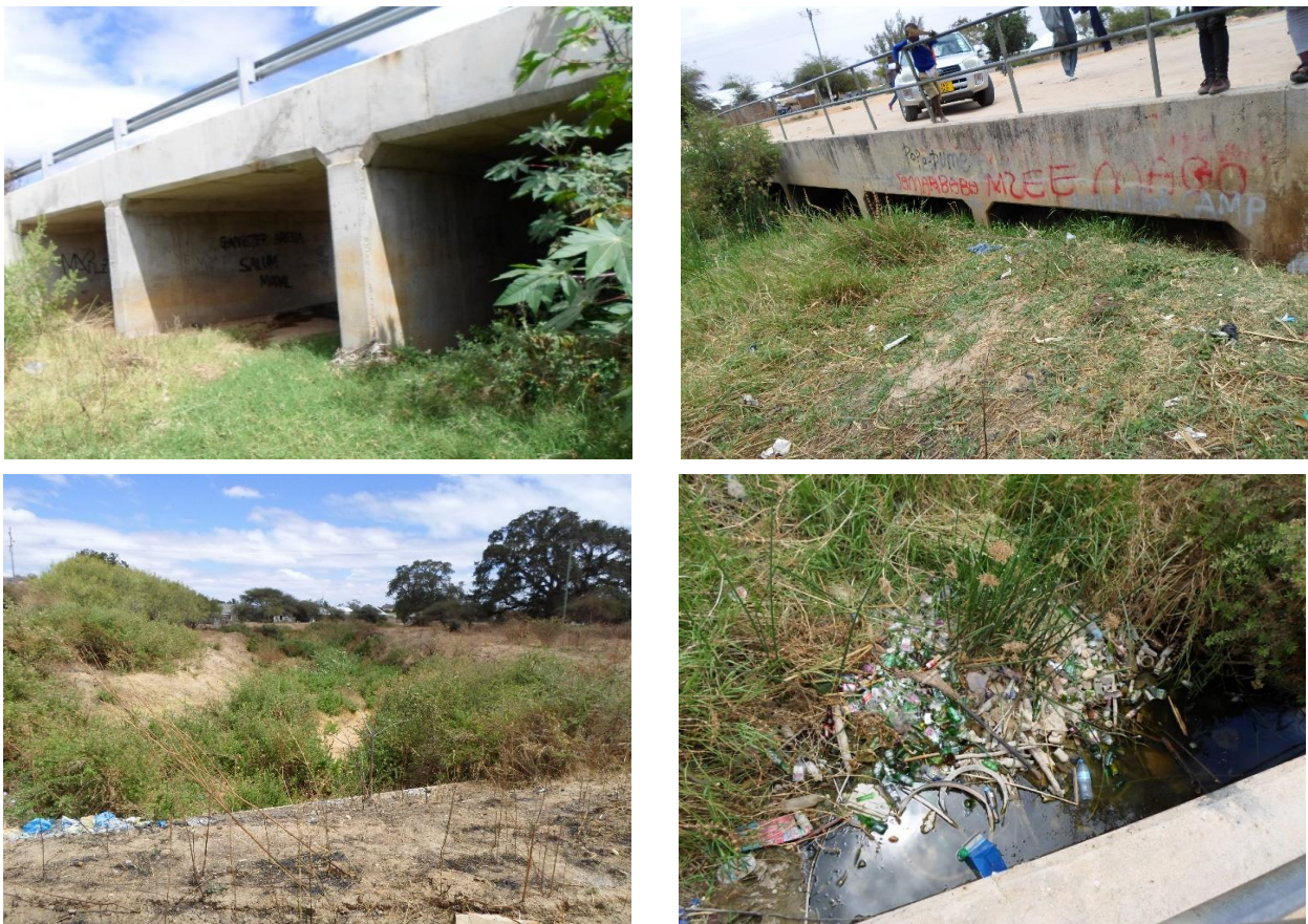
Fig. 23 Kikuyu Storm Water Drain
