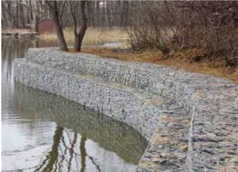
Fig. 39 Gabion for Control of Bank Erosion in Storm Water Drainage
