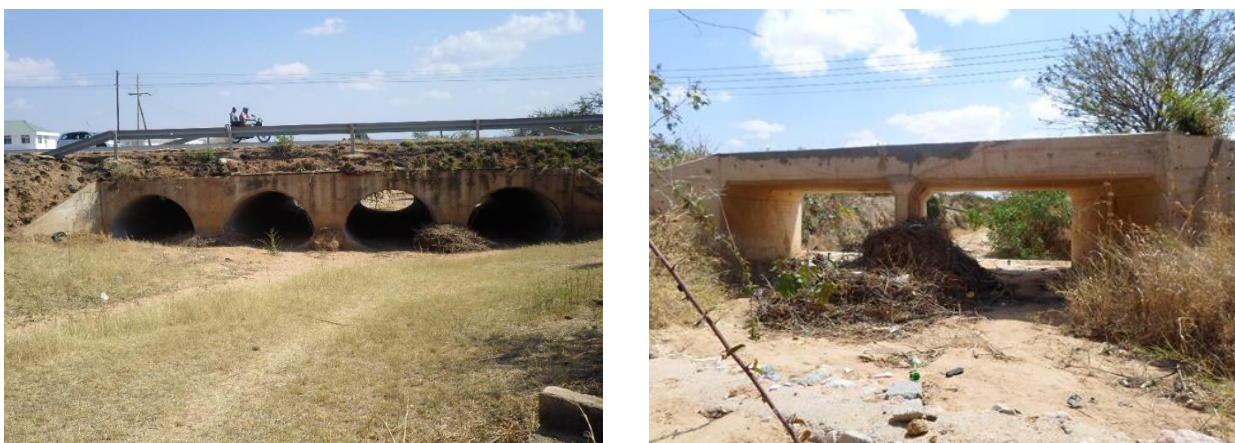
Fig. 21 Mwangaza Storm Water Drain
