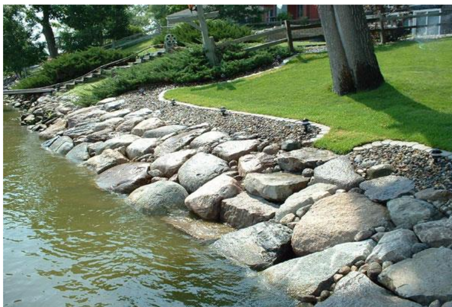
Fig. 40 Riprap Construction for Erosion Prevention in Storm Water Drainage
